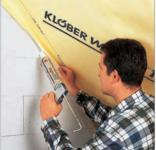
Wallint® 10 eco is a diffusible 2-layer air- and vapour barrier helping to improve the interior climate. Especially for timber boarded roof constructions or any boarded constructions without the use of counterbattens Wallint® 10 eco reveals its strengths. Due to its special coating Wallint® 10 eco prevents the ingress of humidity of the room into the insulation simultaneously offering a high degree of drying capacity and is CE-certified.
